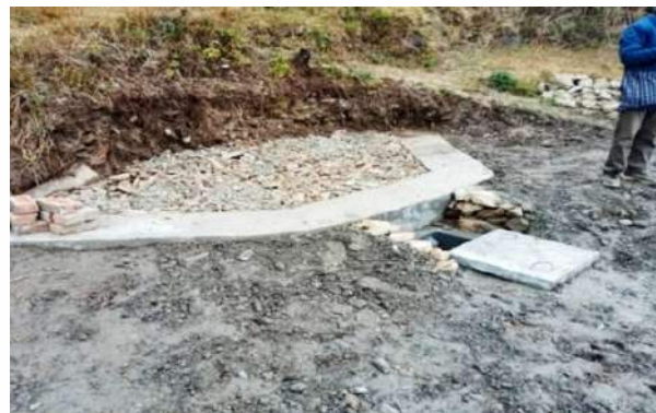
Figure 35: Structural Restoration of the Spring | Source: CHIRAG
