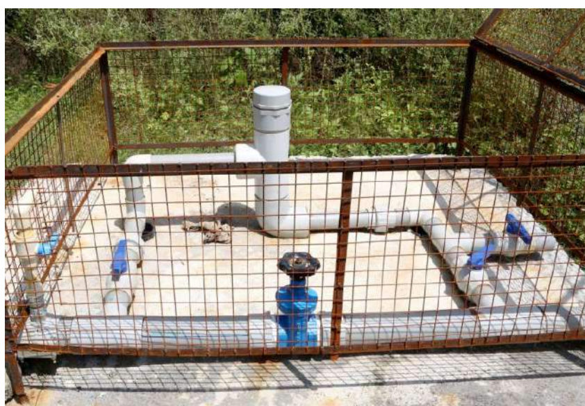
Figure 50: Table-based doser In-Line Chlorination device set up by Evidence Action Source: Evidence Action
