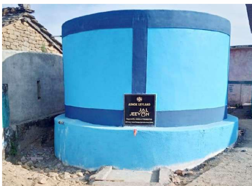
Figure 33: Rainwater Harvesting Tank at Patrani Inter College | Source:CHIRAG
