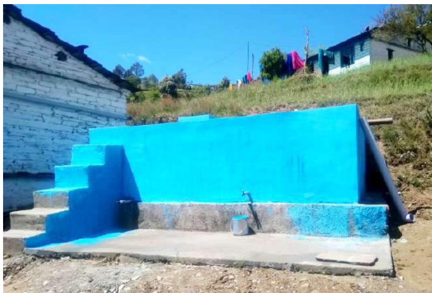
Figure 37: Rainwater harvesting Tank | Source: CHIRAG
