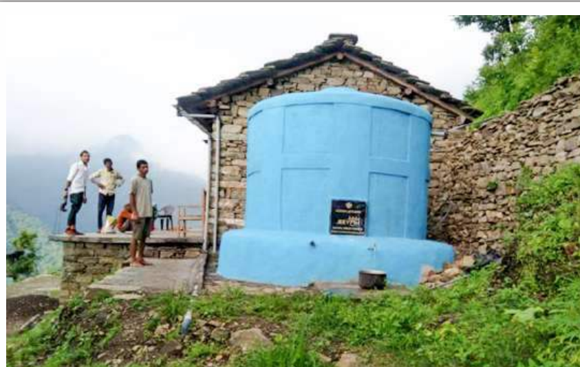
Figure 45: Rain water harvesting Tank | Source: CHIRAG
